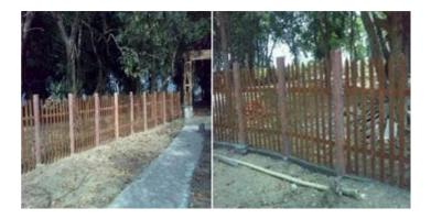
FRP fencing is the ideal replacement of wood fencing & M.S. fencing. FRP fence has advantages of safety, strong, durable, rich color and environment friendly.
